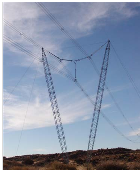
Figures 4.7 and 4.8: Self-supporting Suspension and Strain Tower (left) and Compact Cross Rope suspension Tower (right)
